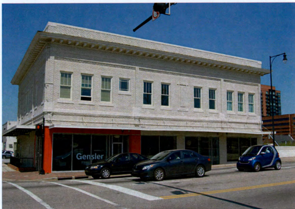
Plate 115. Commercial Block, Front (South) Elevation, Looking North.
