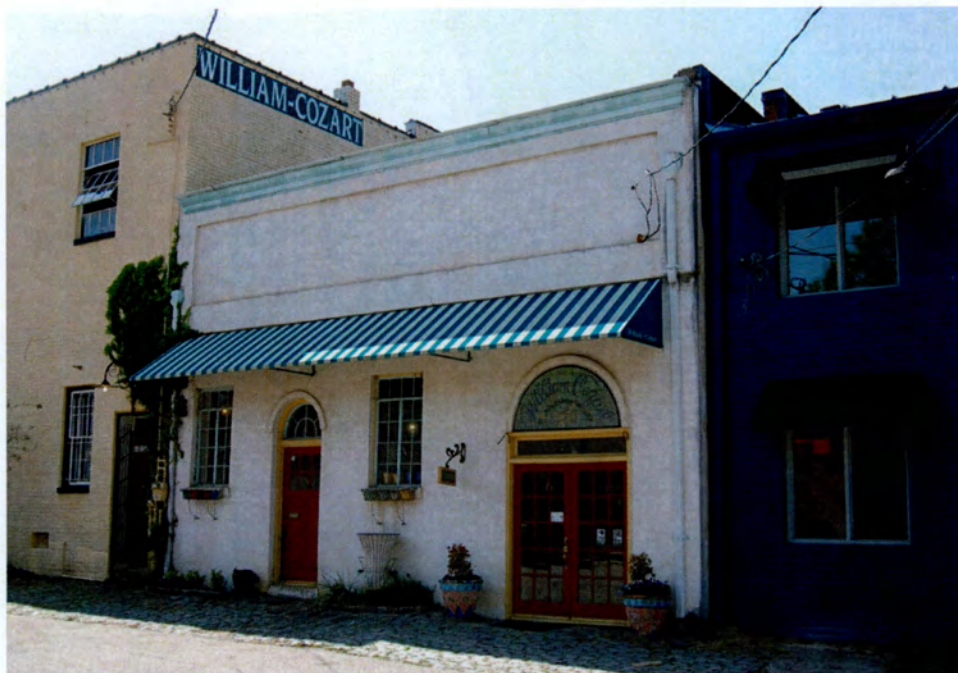
Plate 3. Depot Historic District, Warehouse (No. 21), Looking West.
