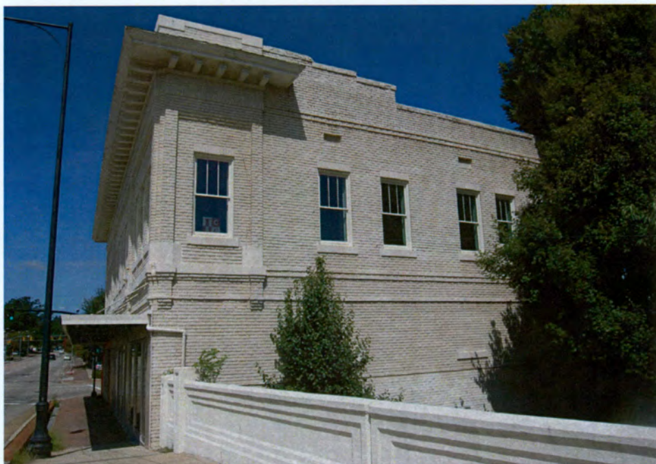
Plate 117. Commercial Block, Side (East) Elevation, Looking West.
