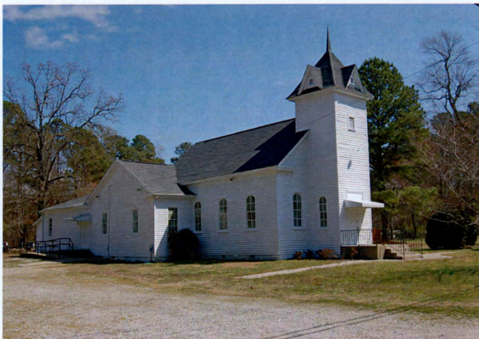
Plate 99. Auburn Christian Church, Looking Northeast.
