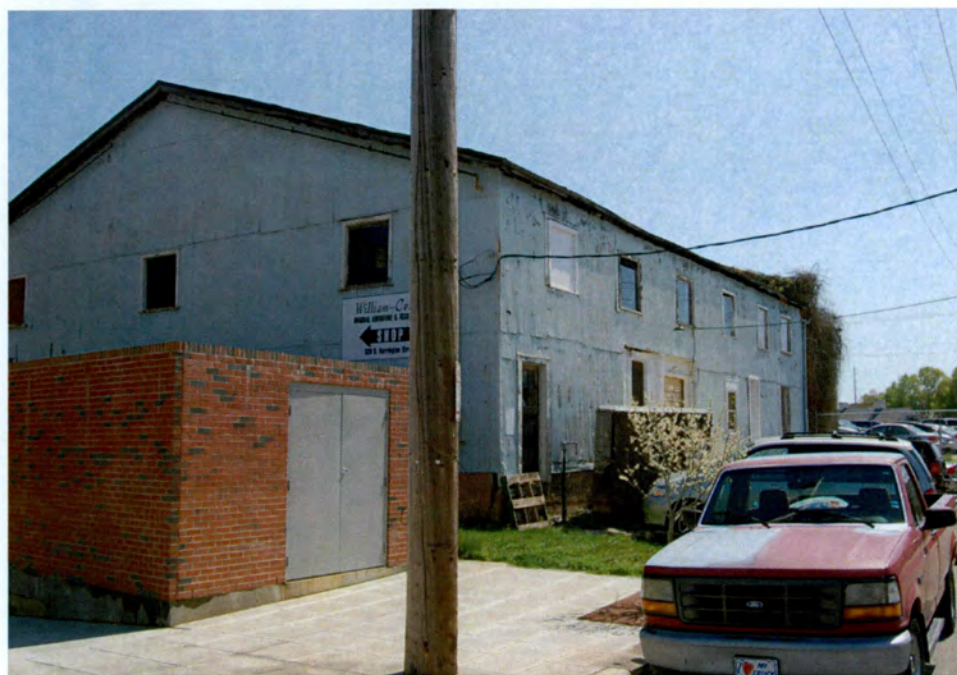
Plate 2. Depot Historic District, Warehouse (No. 20), Looking South.
